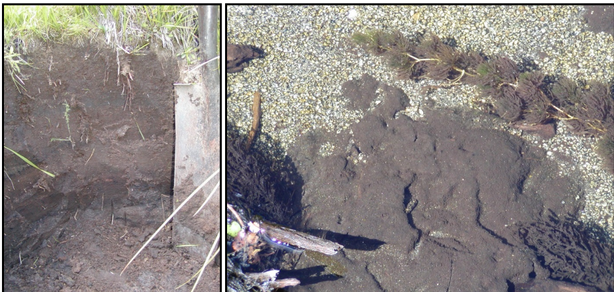
Figure 11a. Left panel: Section of peat streambank adjacent to incised stream channel. This stream channel is a small tributary to the nearby main stream and was not actually flowing at the time. The material in this cut is largely fibrous, compressed peat. Faint blackish zones contain charcoal. Shovel blade is 40 cm long, and section depth is approximately 50 cm. The water table in the channel of the adjacent stream was approximately another 30 cm down or about 80 cm below the surface of this cut. Earlier in the season this channel contains water.
