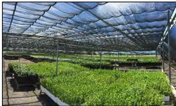
Figure 1: 120'x120' Cravo shadehouse with retractable roof filled with container stock.
