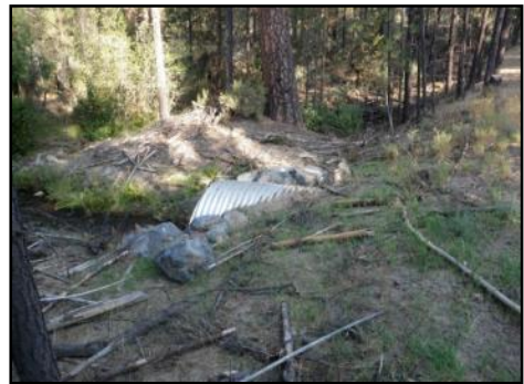
Culvert replacement site one year after planting.
