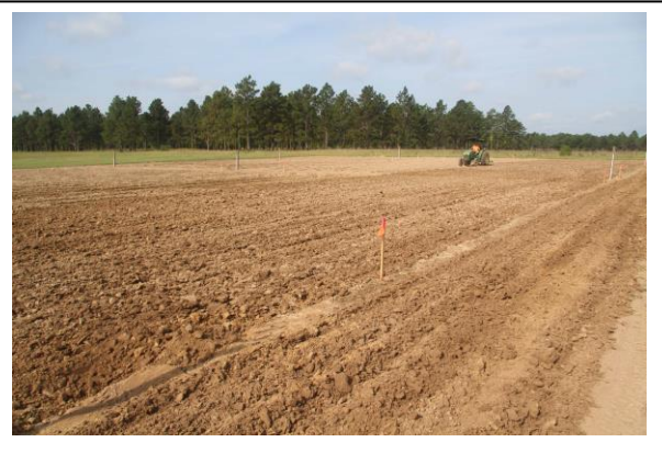
Clean site with irrigation installed – no herbicides used for site prep.
