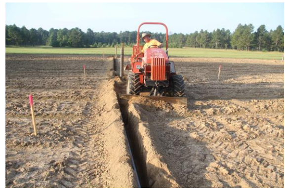
Irrigation installation with assistance from NRCS..
