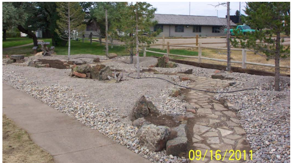
Phase 1 garden construction completed Sept. 2011.
