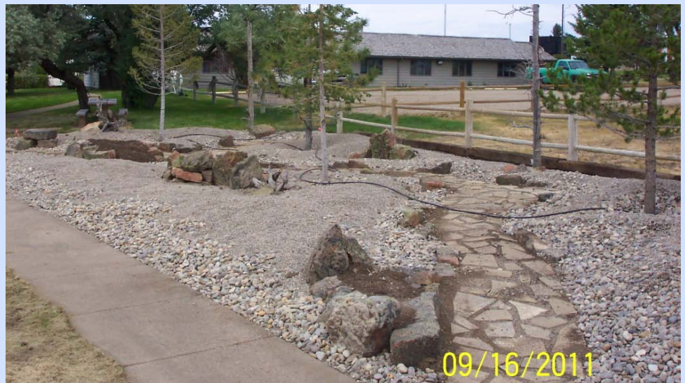
Phase 1 garden construction completed Sept. 2011.
