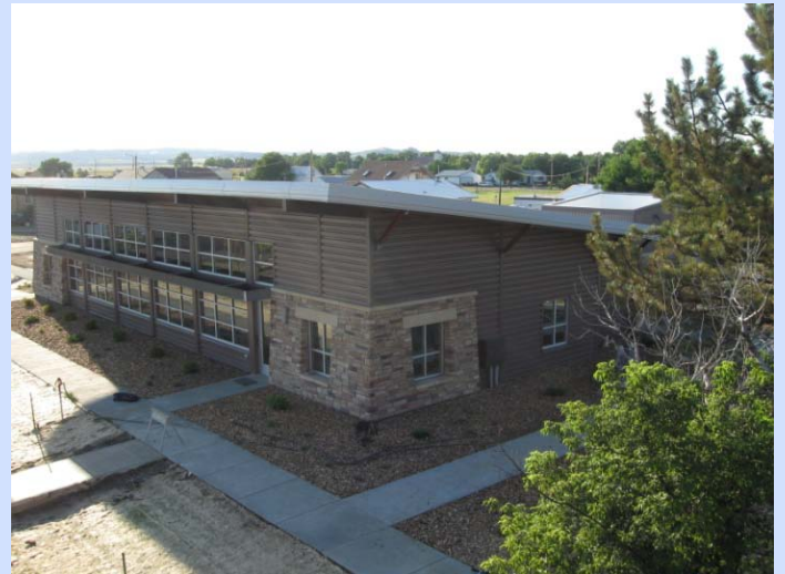
Landscaping finished. August 2011
