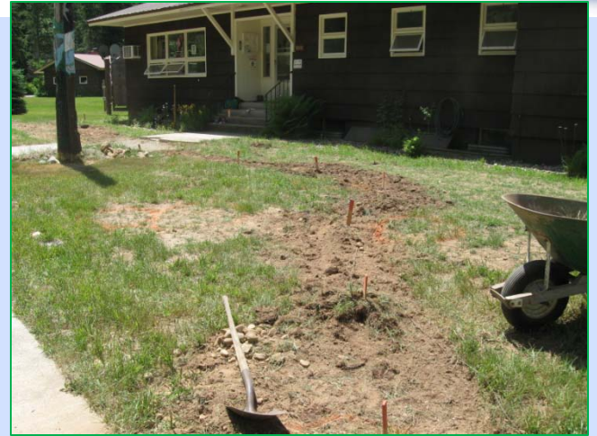
Work begins on the dry creek bed, July 2010
