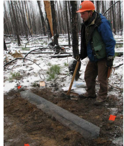
Figure 1. Installation of hardware cloth cages to protect against rodent damage.
