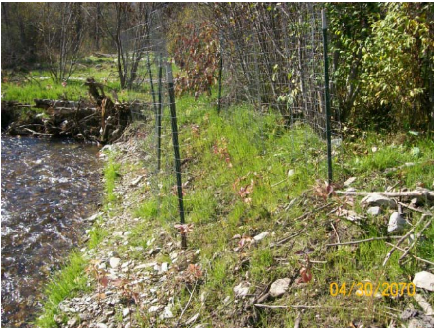
Figure 2. Willow and dogwood plug planting including fencing protection
