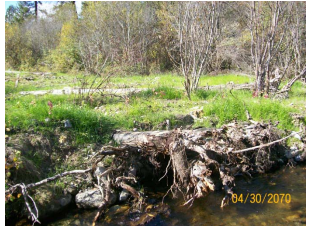
Figure 1. Rootwad placement to protect streambanks and create fish habitat.
