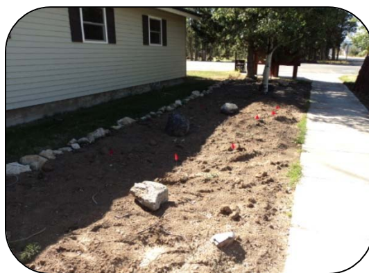
Turfgrass and junipers removed. Irrigation and rock materials placed.
