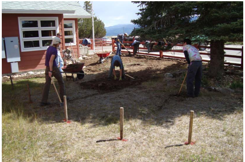
Figure 1. The beginning of project involved removal of the existing lawn.
