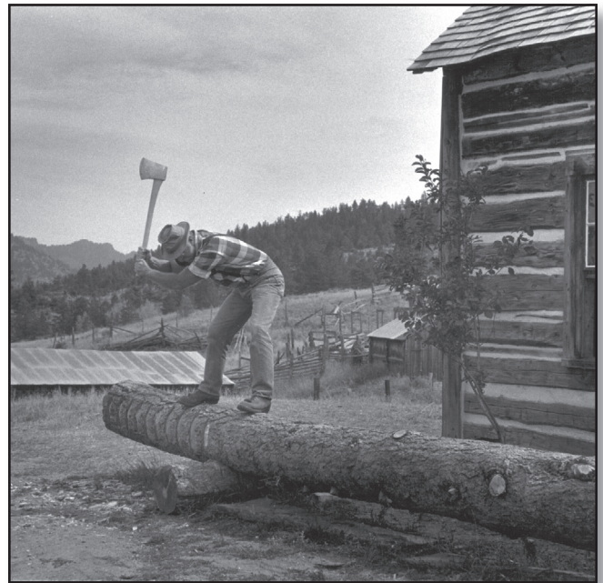
Figure 101—In the scoring technique called juggling, you cut a shallow V-notch down to the depth of the chalk line. Slash scoring is a different technique that doesn't involve cutting a V-notch.
