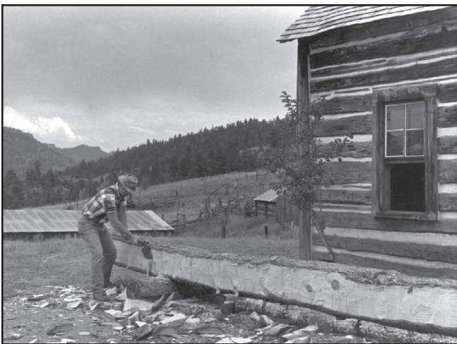
Figure 103—Hew down to the chalk line, removing the excess wood left after scoring.
