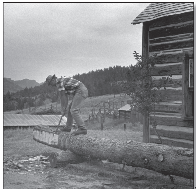
Figure 102—Finish the juggling process by removing the excess wood between V-notches with a single-bit ax.
