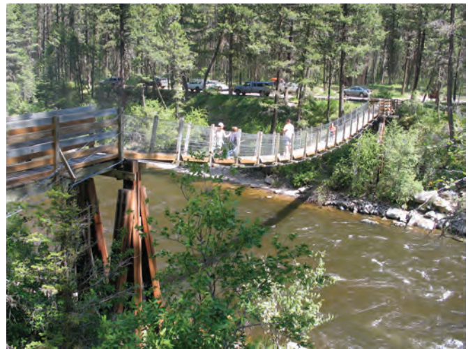
Figure 7—A deck cable bridge supported by two main cables on timber towers.
