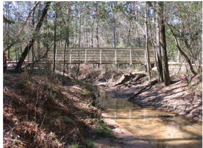
Figure 5—A fiber-reinforced polymer bridge where the truss is also part of the handrail system.
