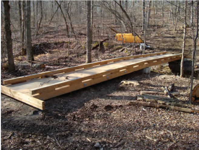
Figure 4—A single-unit bridge with two timber slabs.
