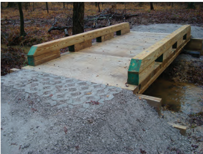
Figure 1—A 15-foot span timber bridge classified as a minor trail bridge, which was constructed using Forest Service standard trail bridge plans.
