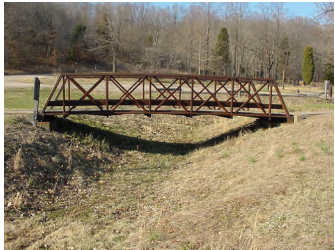
Figure 13—Prefabricated steel bridges are included in the standard trail bridge plans and specifications.
