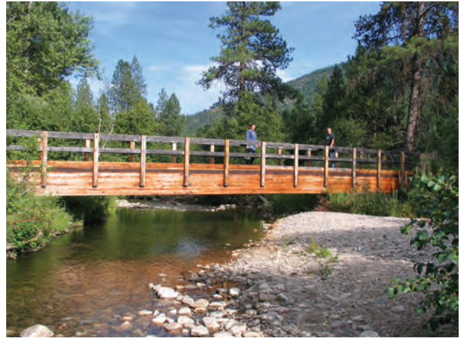
Figure 3—A glued-laminated (glulam) deck girder trail bridge.
