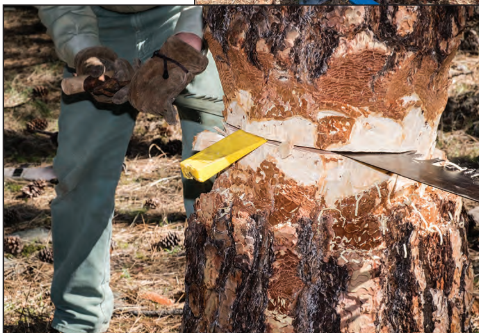
Figure 11–45—Placing a wedge lightly in the kerf of the tree will help alert you when the tree begins to fall.
