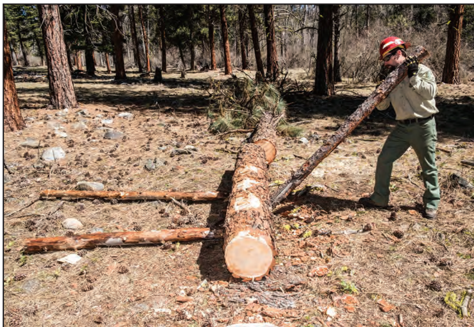
Figure 11-64—Using a lever to move a log.
