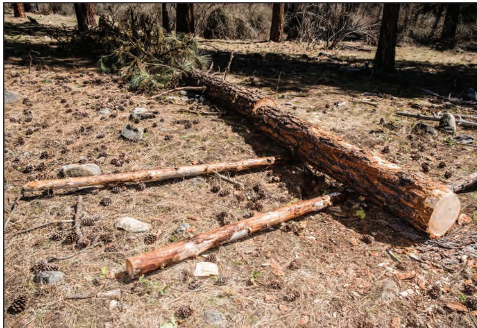
Figure 11–61 —Using poles to roll or skid a cut log out of the way.
