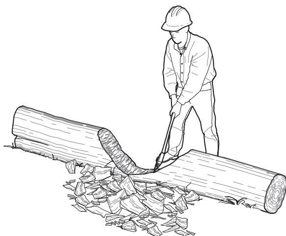
Figure 11–22—Using a horizontal chop to remove the center section between two notches; this is more efficient on larger logs.
