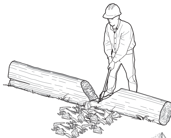
Figure 11–23—Rechopping the side of a notch to widen it; this is more efficient on smaller logs.
