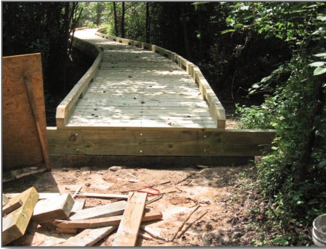
Step 10—Backwall planks installed at the end of the boardwalk keep dirt from sloughing between the beams and prevent moisture from wicking into the ends of the beams.
