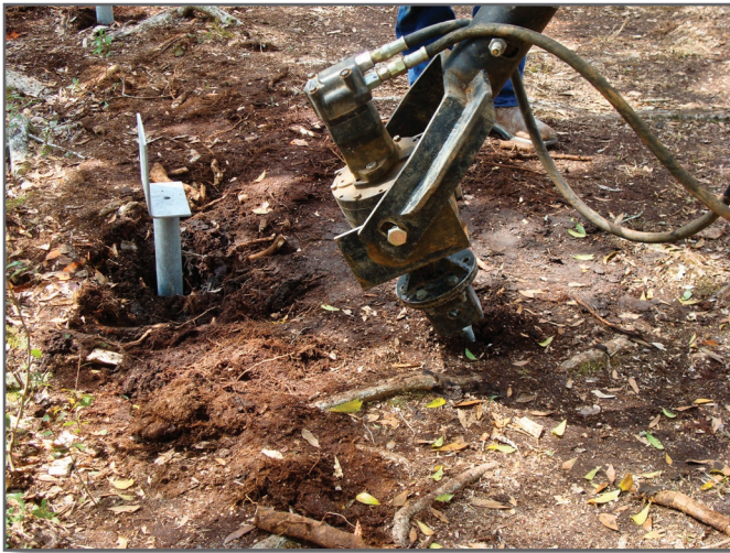
Step 3—Helical piles can be installed vertically or at an angle. Angled installations are especially useful when cross-bracing for lateral support.
