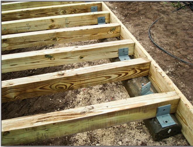
Step 7—The nonelevated end of the structure is secured to a partially embedded plastic curb sill.
