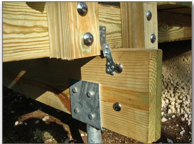
Step 6—Simpson Strong-Tie metal components are used to tie down the joists to the header beam.
