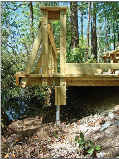
Step 8—The viewing/fishing platform support system.
