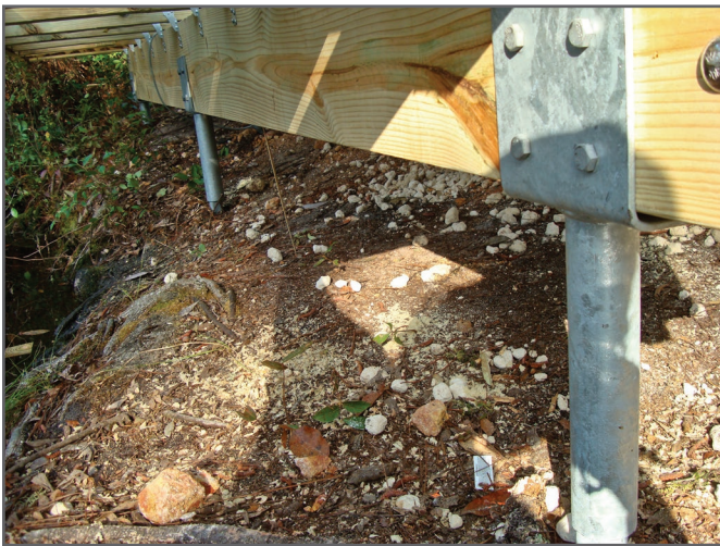
Step 4—Saddle brackets are bolted to helical piles to support the header beam, forming a bent. In this case, the timbers are alkaline copper quaternary (ACQ)-treated southern yellow pine.
