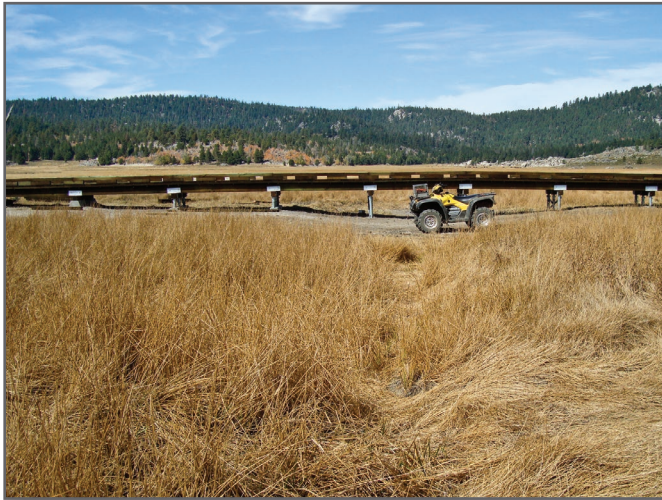
Figure 3—Precast concrete barriers on top of geogrid filled with stone provide solid footing for this Snake Creek Trail boardwalk at the Inyo National Forest in California.
