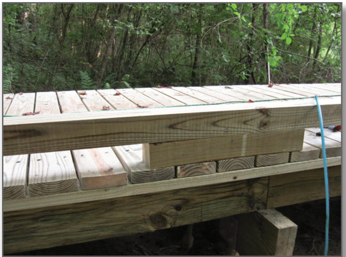
Step 9—Curbing (6 inch by 6 inch or 4 inch by 4 inch, depending on the width of maintenance equipment using the boardwalk) on top of scupper blocks is specified in lieu of railings for this OHV trail.
