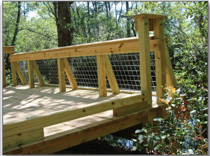
Step 9—The front handrail is sloped to allow the legs and front wheels of a wheelchair to be positioned slightly underneath the top rail. The handrail height is 34 inches. Welded wire mesh is installed to discourage alligators from using the platform, to provide better views of the canal channel scenery, and to prevent small children from falling in the water.
