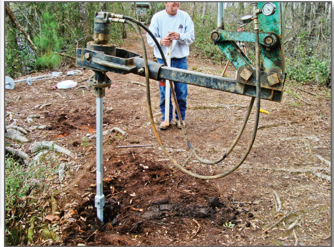
Figure 4—Specialized equipment is needed to install helical piles. For this installation, Trails Unlimited installed 12 helical piles for 4 viewing platforms in 4 hours.
