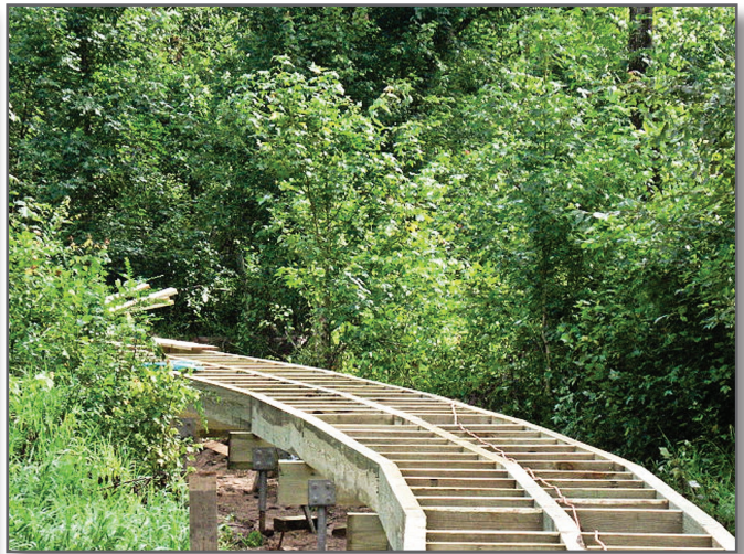
Step 8—Bracing is added between the stringers to prevent the stringers from rotating.
