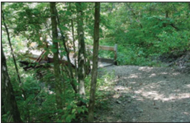
Figure 34—This alignment causes a blind spot for oncoming traffic.
