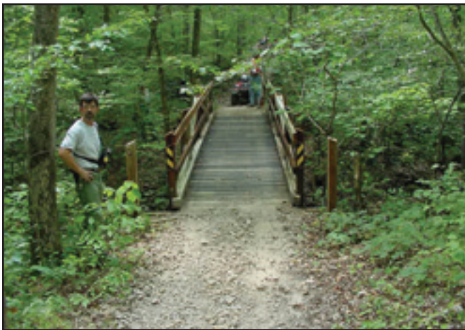
Figure 33—This bridge is on a good alignment that allows OHV riders to see oncoming vehicles.
