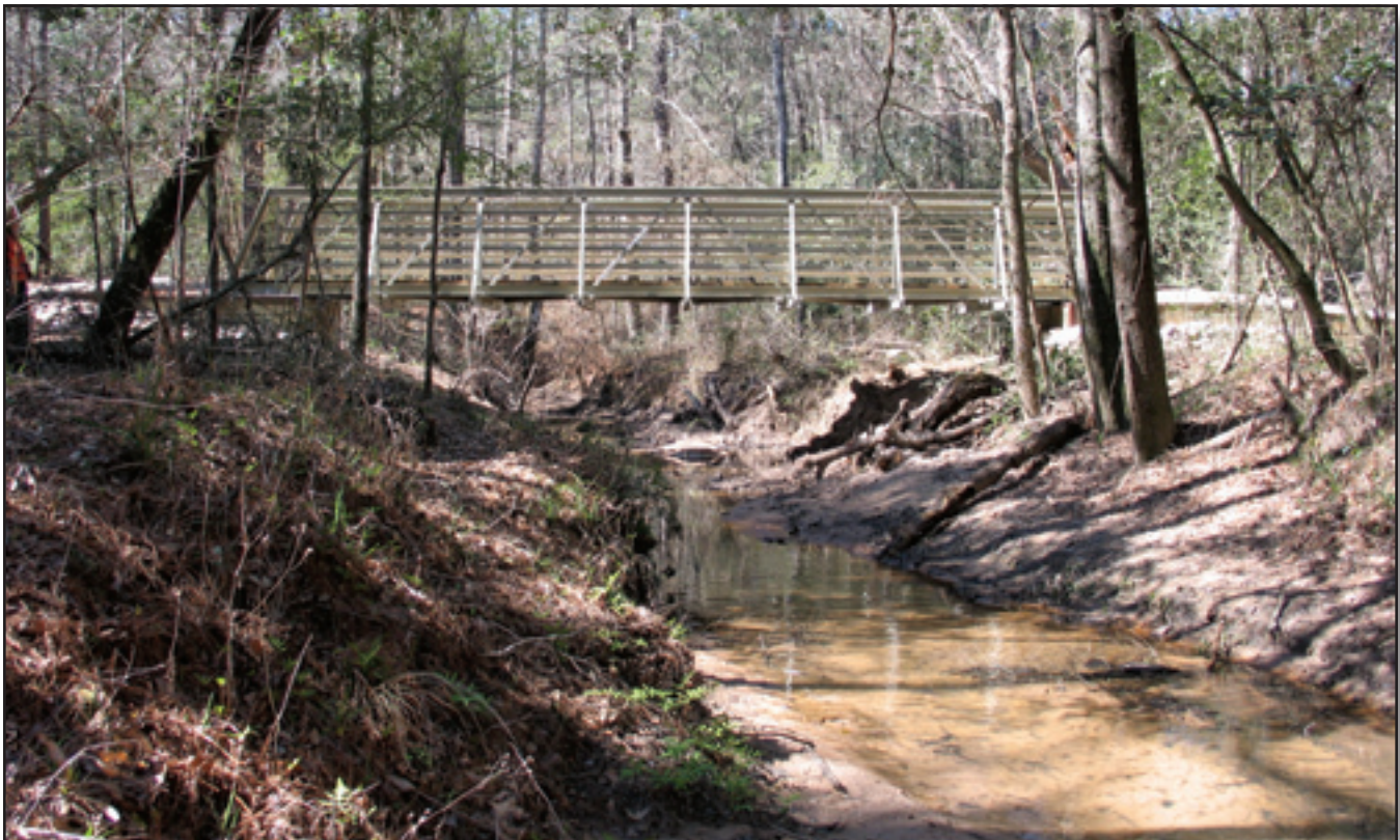
Figure 1—A new fiber-reinforced polymer trail bridge in the Sam Houston National Forest.
