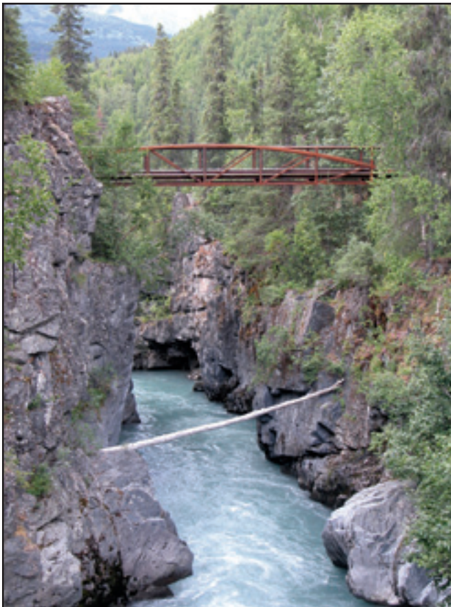
Figure 21—This bridge is set high to allow rafters to pass underneath.
