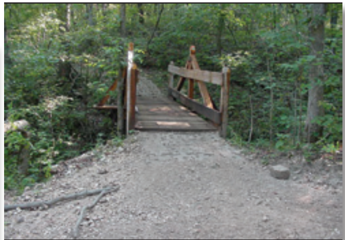
Figure 35—This bridge has a slight grade, allowing water and debris to run off the bridge deck.
