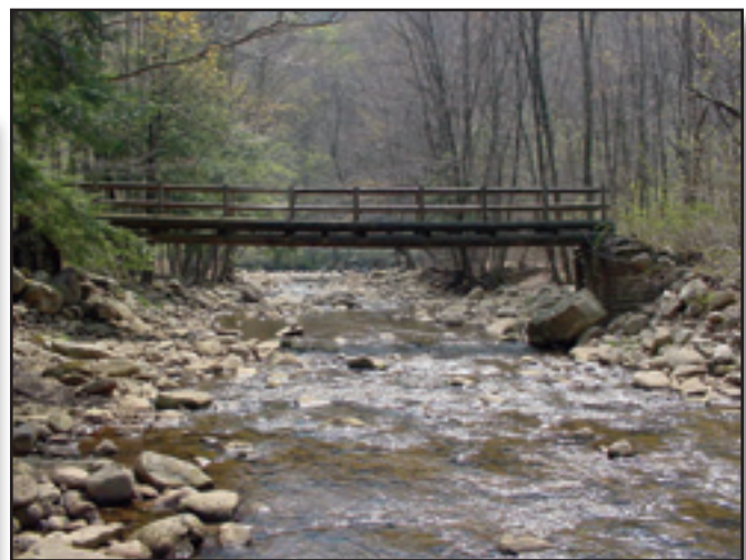
Figure 16—This bridge is on a side stream and in a flood plain. The back-water effect during floods on the main stream has floated this bridge away twice.
