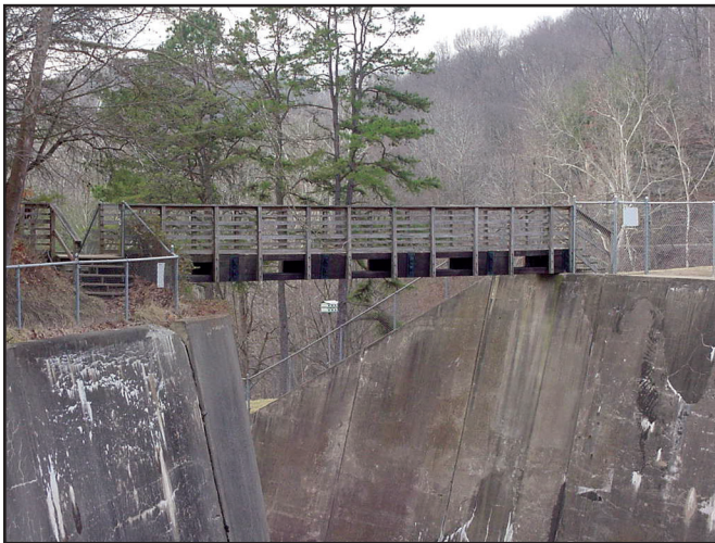
Figure 5—Some sites are very simple and require only minor site investigation.
