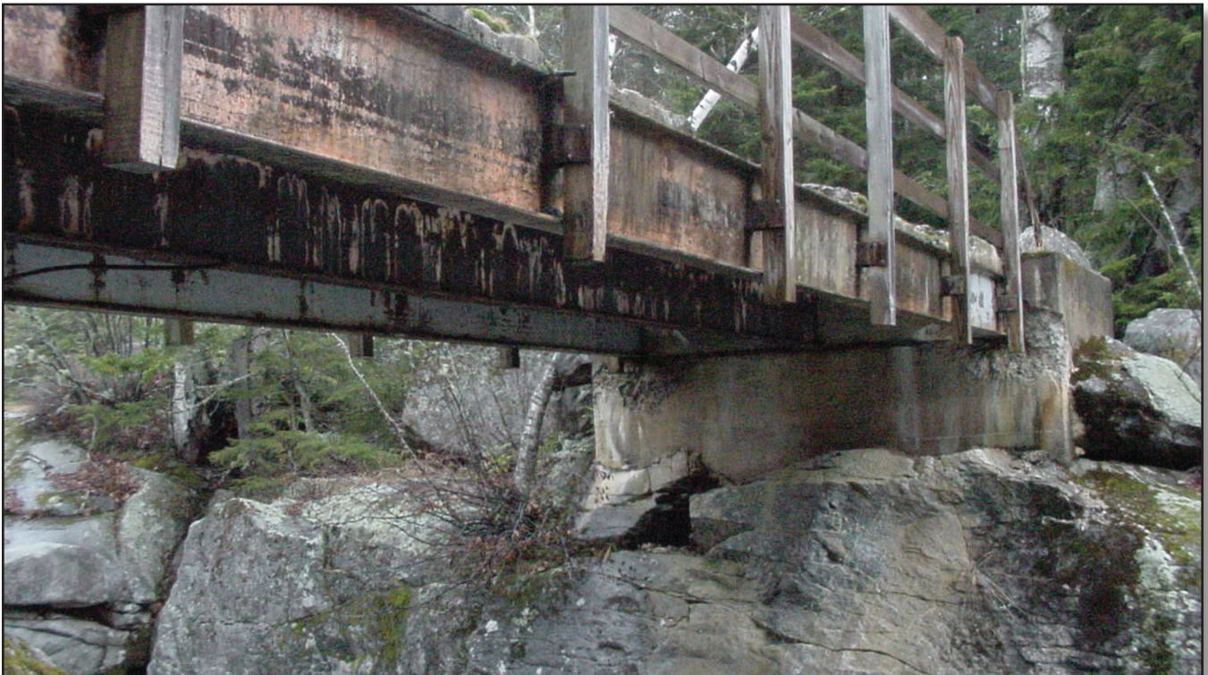
Figure 19—A bridge abutment placed on a bedrock streambank.
