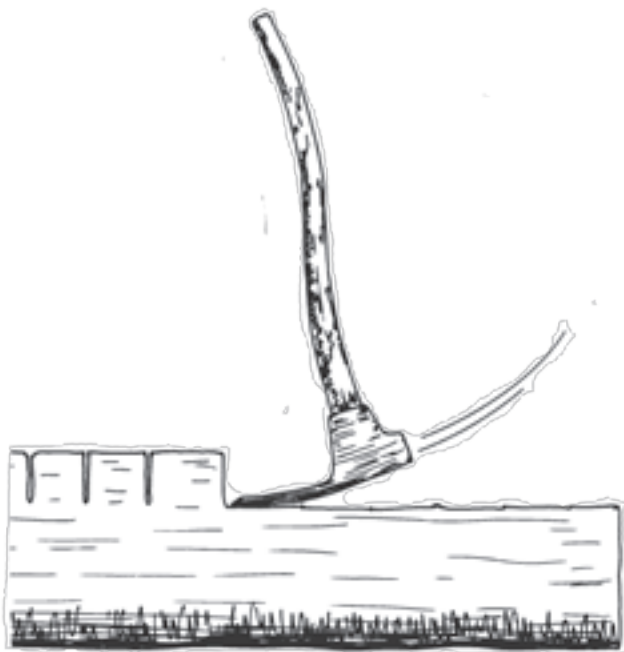
Hewing a log with a carpenter's adze.
