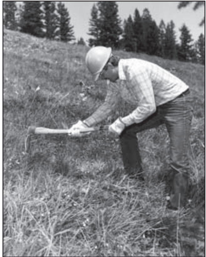
Grub hoe being used for trail work.
