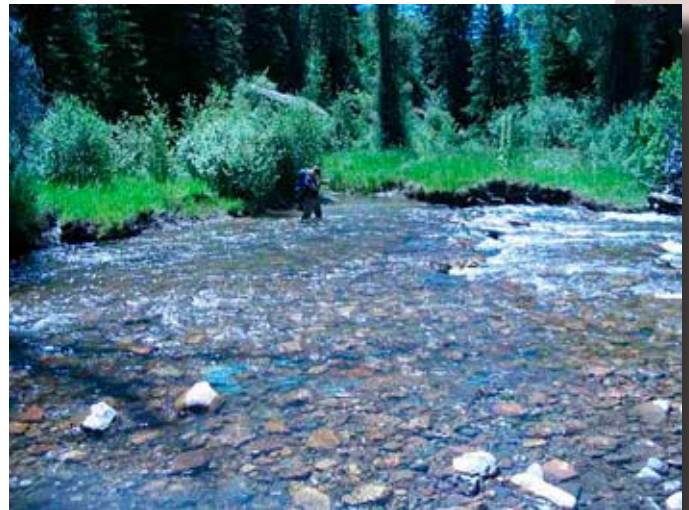
Stream margin diversion without water control structure—Battle Creek, Medicine Bow NF. The diversion dam is reconstructed every year from rock in the channel (Photo by Dave Gloss.)
