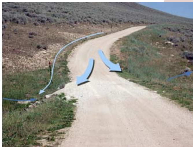
Figure 13. Identifying the surface drainage pattern is a key indicator in the SWRCI form.
