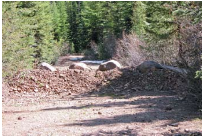
Figure 12. Boulder barricade used to restrict vehicle access
