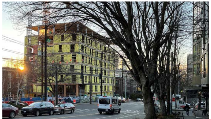
The first Type IV-C building of its kind, Seattle’s Heartwood tops out at eight stories. Courtesy photo by atelierjones, llc.
