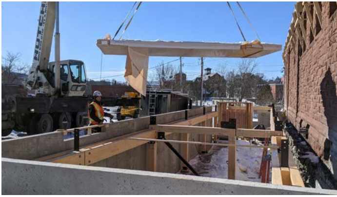
First-of-its-kind eastern hemlock CLT panel installed at the Fairbanks Museum. Courtesy of Innovative Natural Resources Solutions, LLC.
