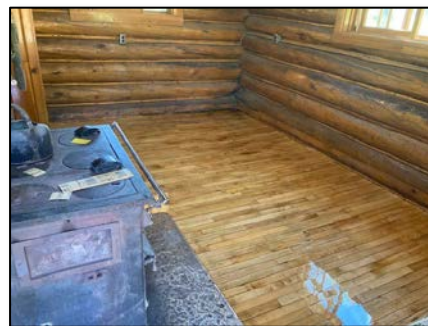
The floor shines following sanding and refinishing at the Birch Creek cabin
