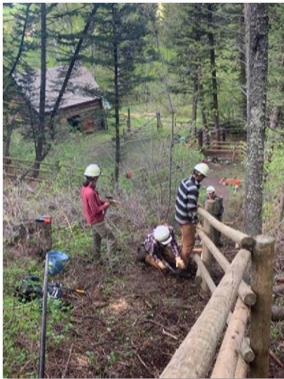
Recreation crew hard at work on stock fencing at the Bear Creek Campground
