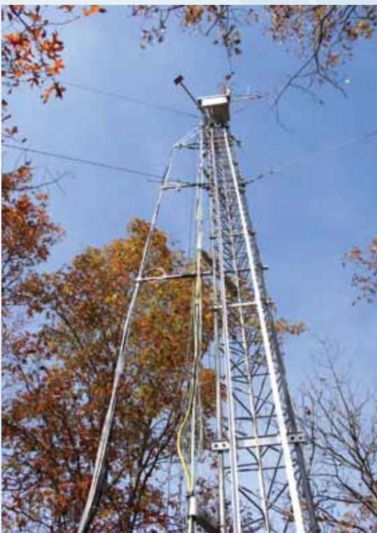
Figure 2. Mitigation of climate change impacts: Monitoring forest carbon exchange with eddy-flux towers, here at Forest Service Northern Research Station facilities in Howland, ME. The towers support the apparatus used to measure the hourly uptake and release of CO 2 by trees and the soil and determine impacts on carbon storage by management treatments over daily, seasonal, and annual growth cycles. Photo from John Lee, University of Maine.
