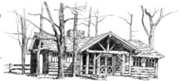
*Indigenous Materials:* This was a heavily forested province (and heavily logged), where logs remained a favored building material into the 20th century. Logs were sometimes left unfinished. The chinking could be removed for summer ventilation. Stone was common, where it could be quarried or collected in fields.
