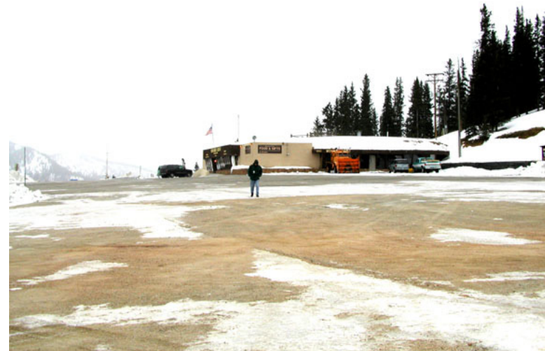
Monarch Pass parking and concessionaire facilities in December 2002
