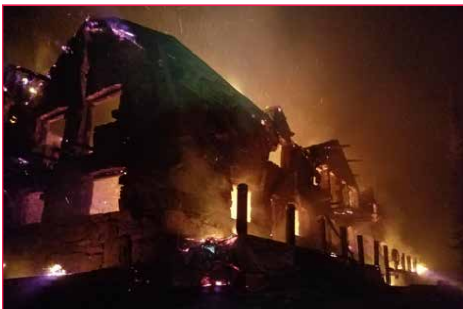
The Sperry Chalet in Glacier National Park being destroyed by the Sprague Fire in 2017. Source: Inciweb (2017); photo: National Park Service.
