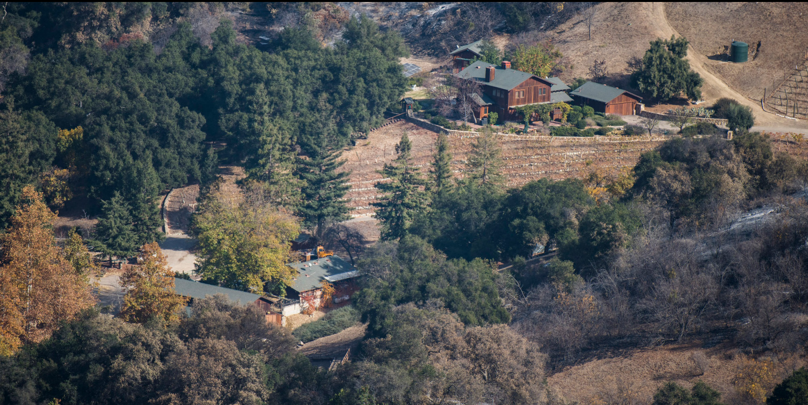
Damage from the 2017 Thomas Fire near the Los Padres National Forest in California. Structures survived the fire due to defensible space. Photo: USDA Forest Service, Stuart Palley (December 22, 2017).
