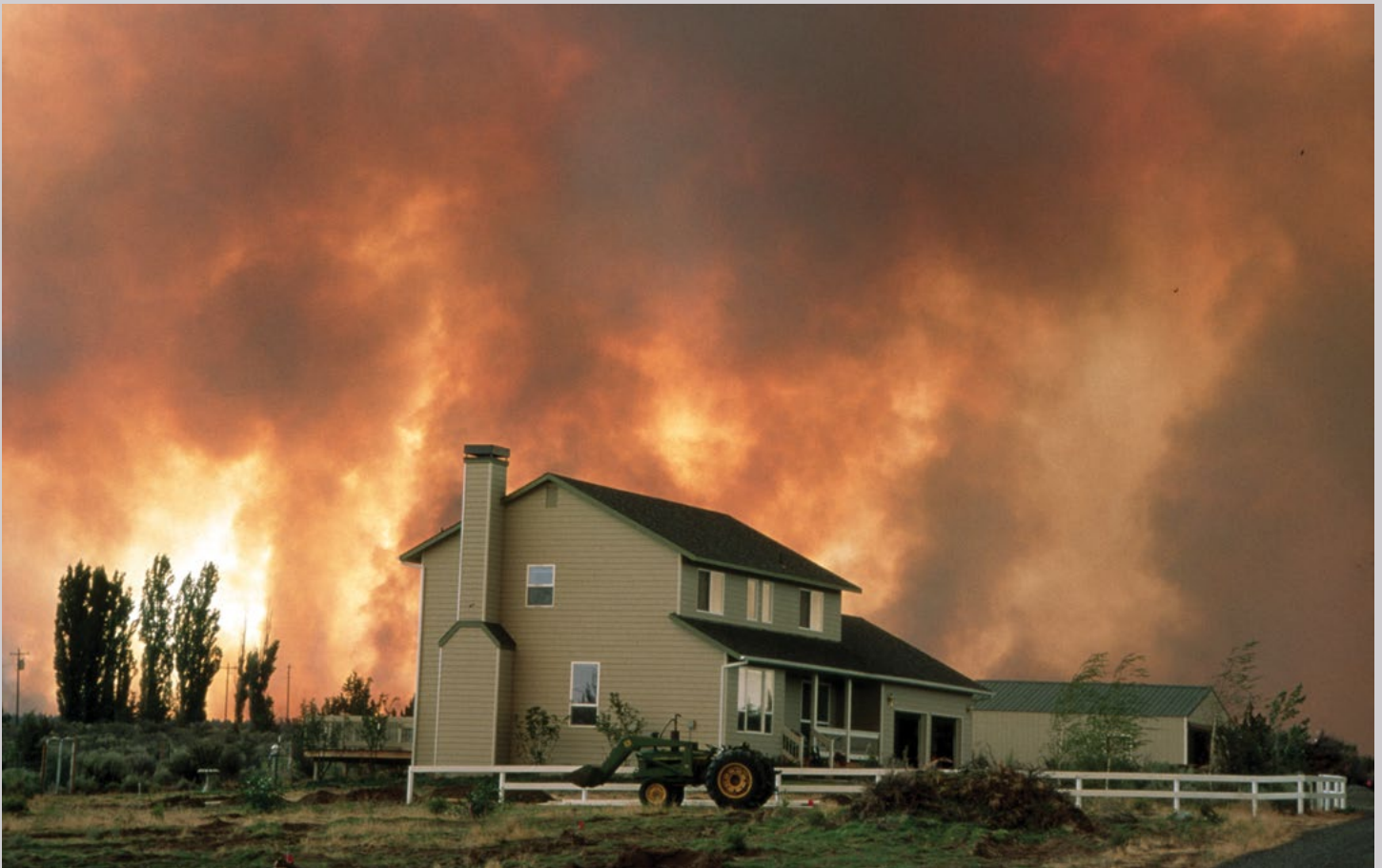
A home in the wildland-urban interface at risk from a wildfire in 2011 on the Deschutes National Forest in Oregon. USDA Forest Service photo.
