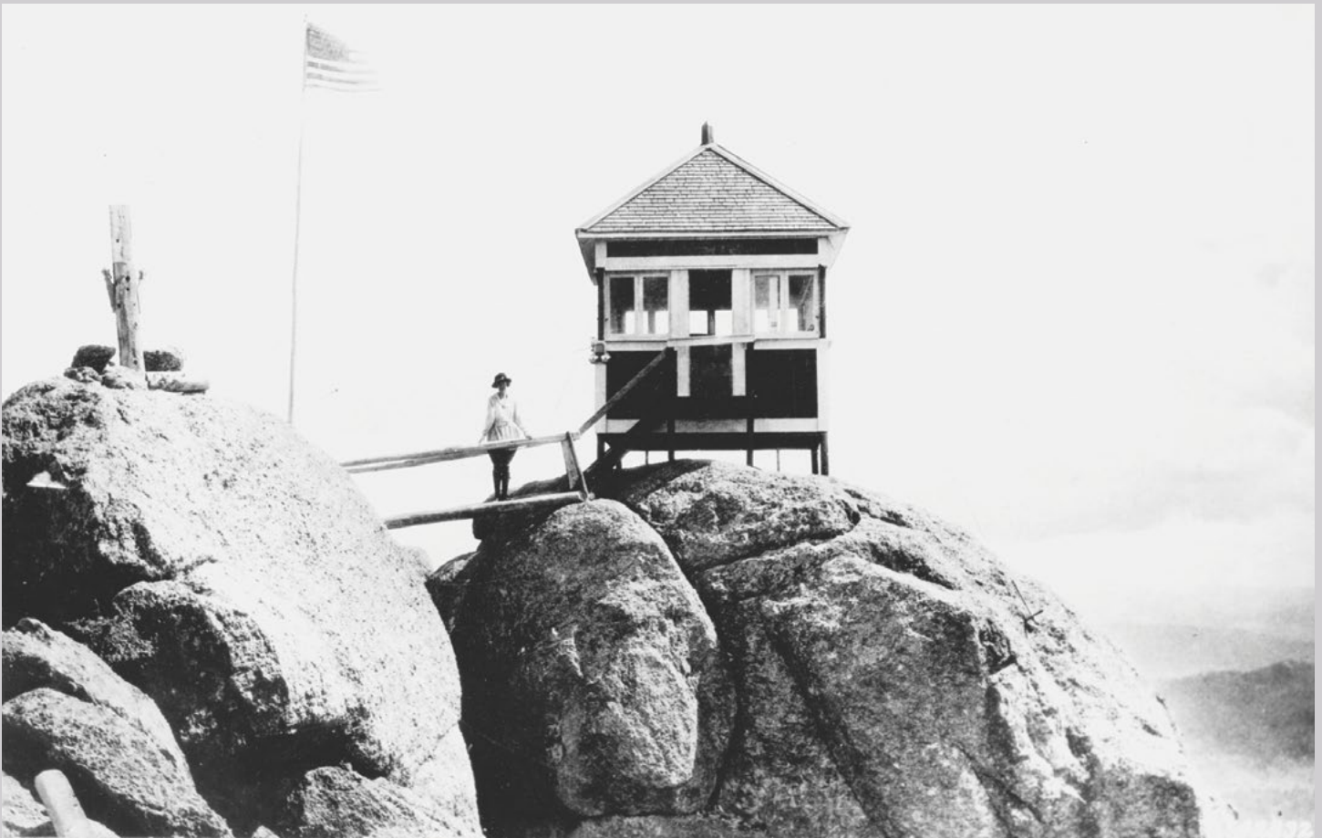
Devil's Head Fire Lookout on the Pike National Forest in Colorado in 1919, with Helen Dowe as seasonal fire lookout. USDA Forest Service photo by F.E. Colburn.
