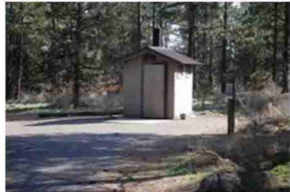
Typical single vault toilet at a trailhead.
