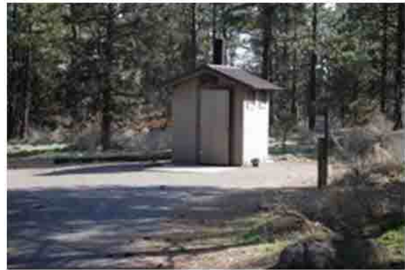
Typical single vault toilet at a trailhead.
