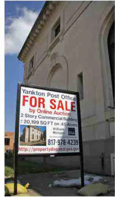
Figure 9. Example of the transfer, lease, or sale of a property out of federal ownership or control. Once a property is out of federal ownership or control, it is no longer automatically subject to Section 106 and the measures to take into account the effects a project may have on that property.
