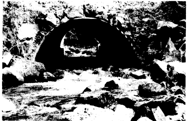
Figure 1.--Pipe arch used to allow fish passage.
