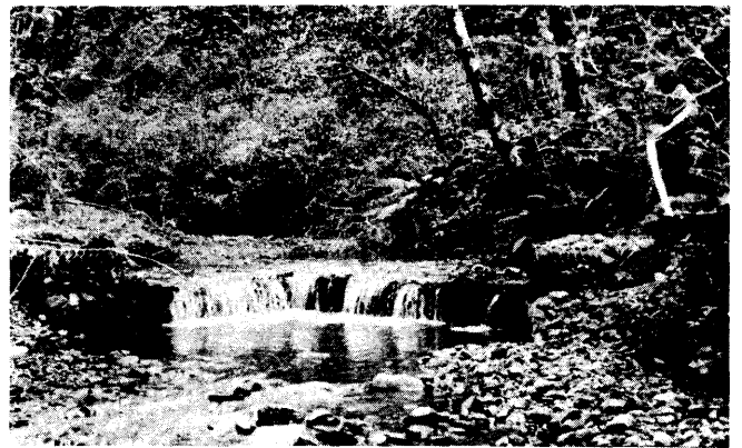
Figure 5.--Reverse V gabion.
