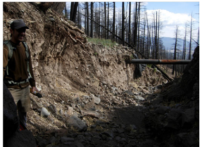
Fig. 12. Deeply incised (3 m) main drainage gully within the Schultz Fire along the Waterline Road, Coconino National Forest, Arizona, USA. (Photo by Karen A. Koestner).
