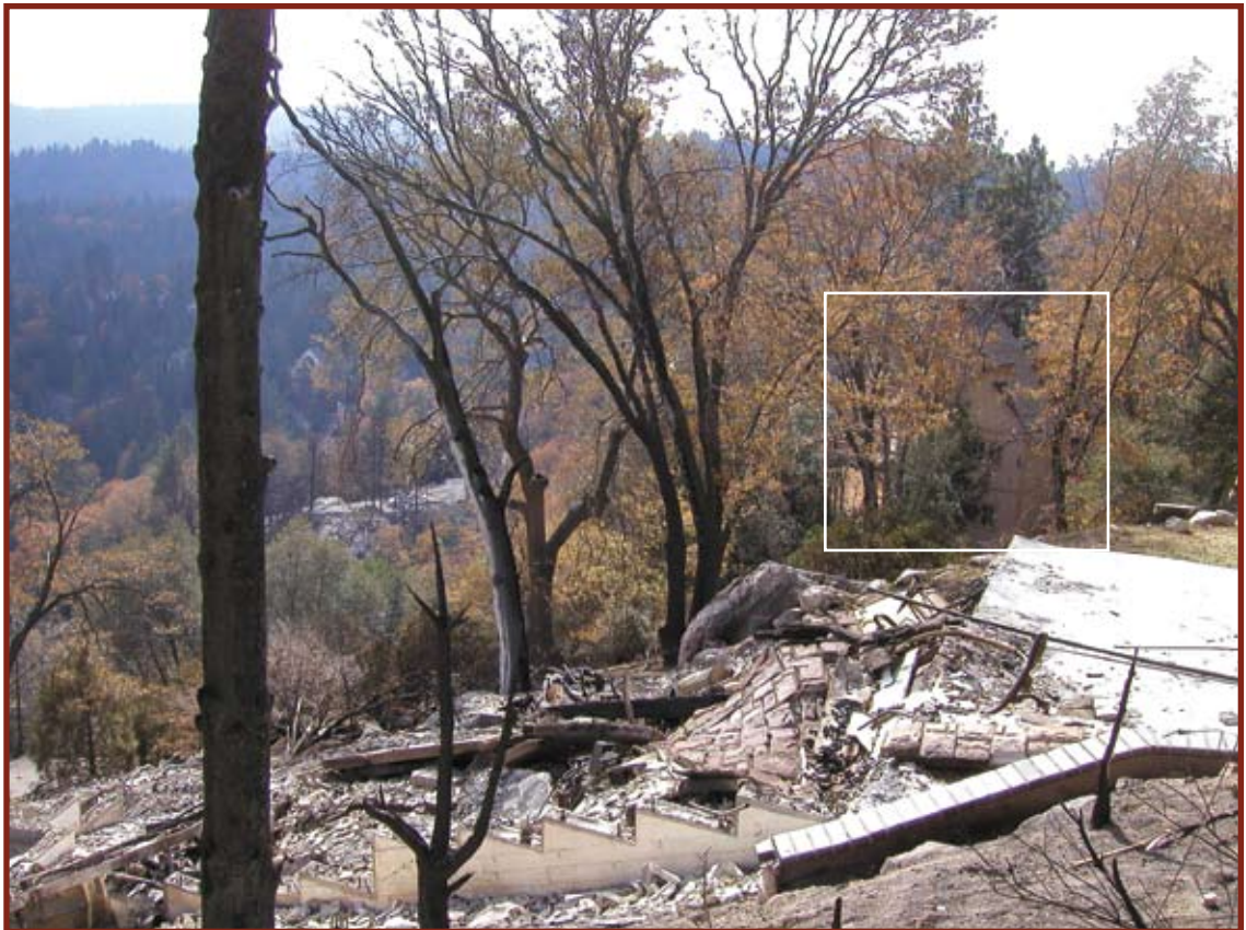
Figure 21. Destroyed homes at 899 and 905 Sonoma Dr. looking southwest through two vacant parcels that surface burned with an undamaged home (framed) in the background (875 Sonoma).
