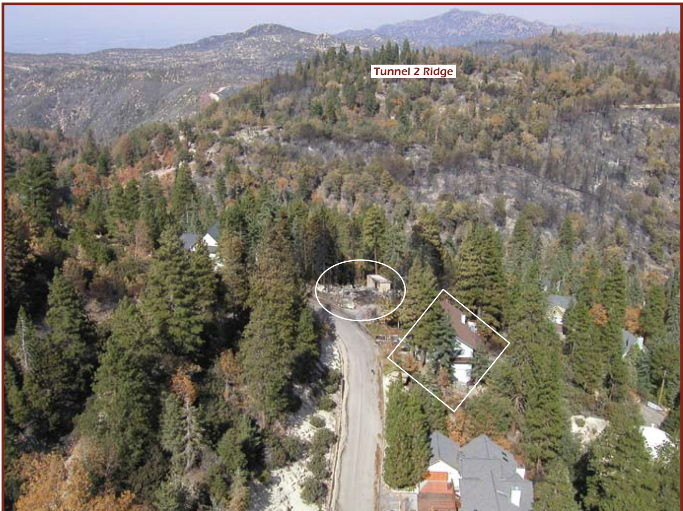
Figure 31. Aerial view looking northwest up Walnut Hills Dr. to destroyed home at 26142 (circled) and damaged home at 26150 (framed). Tunnel 2 Ridge is directly across drainage and shows evidence of group tree torching.
