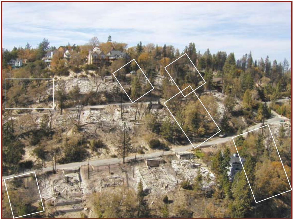
Figure 20. Aerial view facing west with Madera Ln. at the bottom, Del Norte Ln. in the middle, and Sonoma Dr. just below the homes at the top of the hill (Kings Ct.). Note the unconsumed vegetation between the destroyed homes, particularly in the vacant parcels that were burned by surface fire (framed areas).
