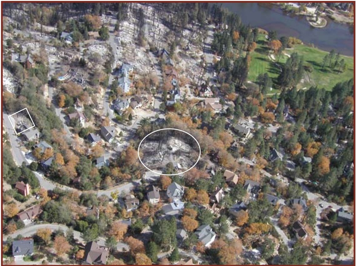
Figure 24. Aerial view looking down on five homes (circled) on Del Norte Ln. and Merced Ln. that were initially started by firebrands, possibly from burning homes or vegetation at 837 or 845 Del Norte (framed).
