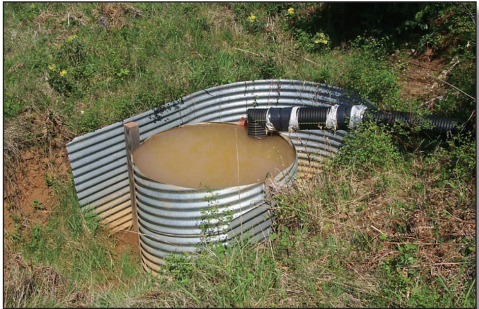
Figure 8 —The upper sediment tank is located on a gravel pod. The lower settling tank is located on a concrete pod behind a steel retaining wall.
