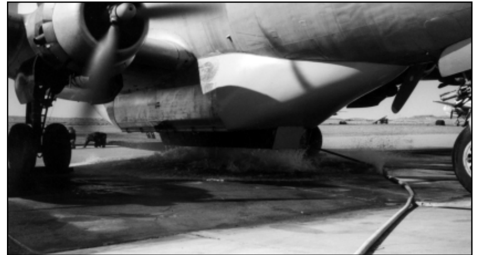
Figure 1—A static test of the Aero Flite DC-4 airtanker.
