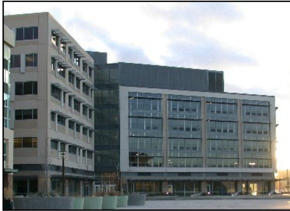
Idaho Water Center
