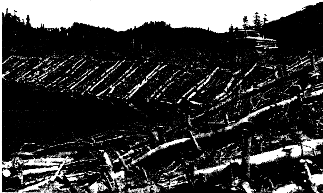
Figure 2- Bank stabilization along Prairie Creek. Willow logs and hog wire were staked to what was a bare, eroding streambank. January 1984.
