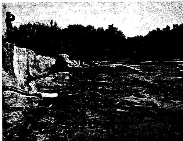
Figure 2.--Bank erosion on San Pedro River south of Winkelman, Arizona.
