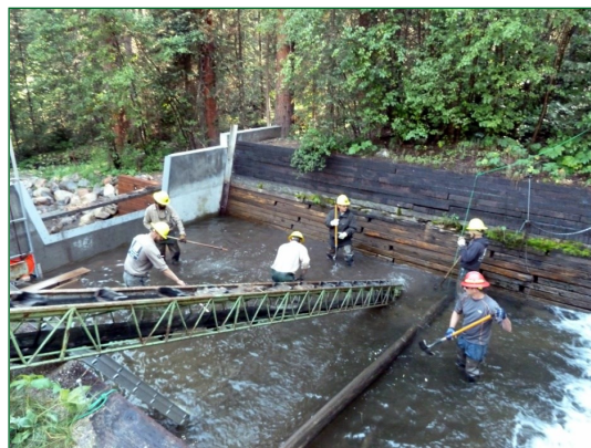
Veteran work crew removing sediment from a weir pond in Fraser Experimental Forest.
