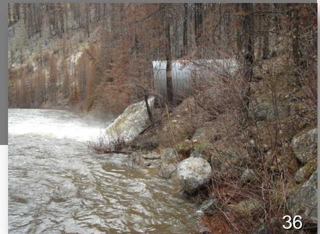
Goat Creek culvert before restoration; high water, Payette NF
