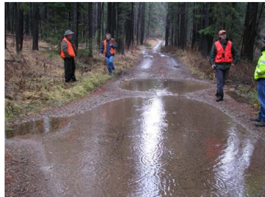
Figure 3: Example of existing ford on South Fork Poorman Creek
