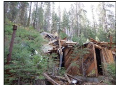
Photo 4: Mill building during removal
