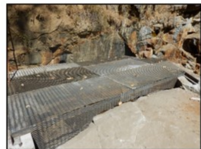
Photo 6: Shaft closed with metal grate
