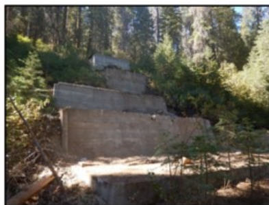
Photo 5: Mill building post-project
