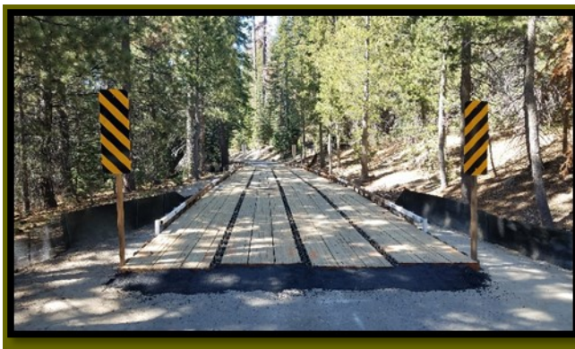
Figure 5.1.1. Elevated roadway segment.
