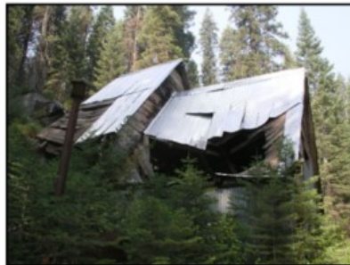
Photo 3: Mill building pre-project
