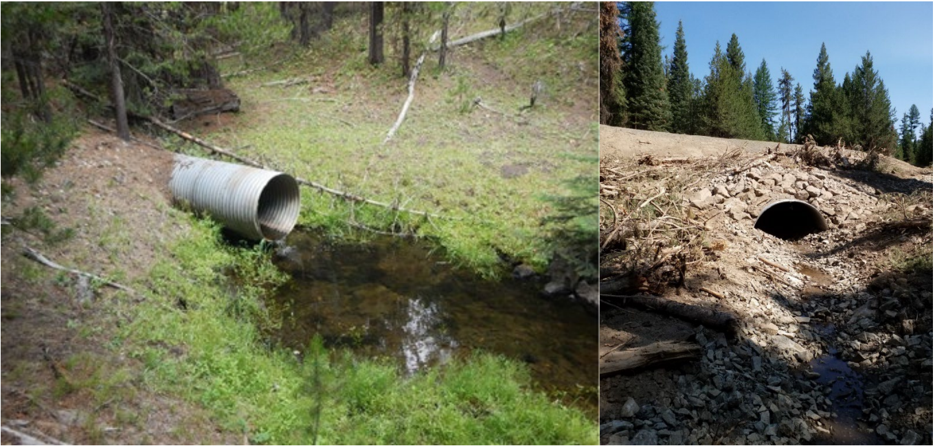
Tinker Creek Fish Passage Photos
