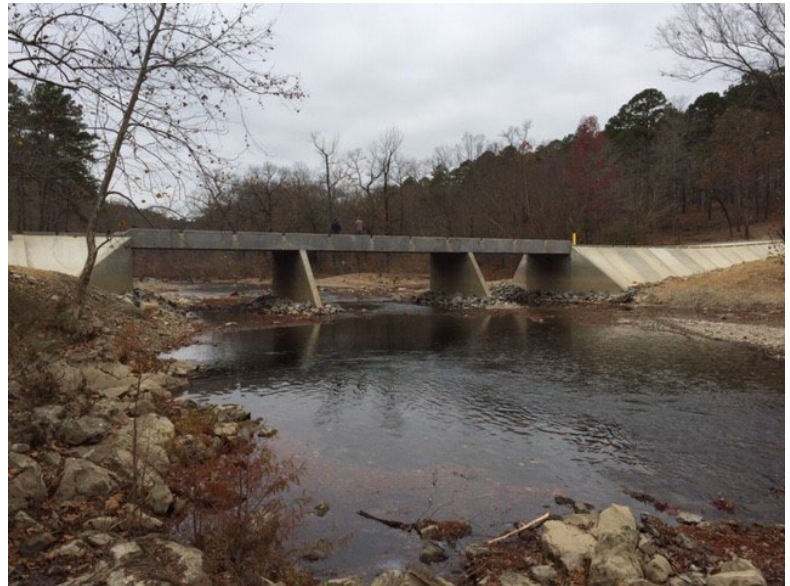
Figure 9. Buffalo Creek crossing within the Shortleaf – Bluestem Community CFLRP project area in Oklahoma, finished in 2021. This project was funded with non-CFLRP dollars in a previous fiscal year, and contribute stable access to a large part of the project area allowing timber, fire, and wildlife treatments, and also making aquatic organism passage possible.
