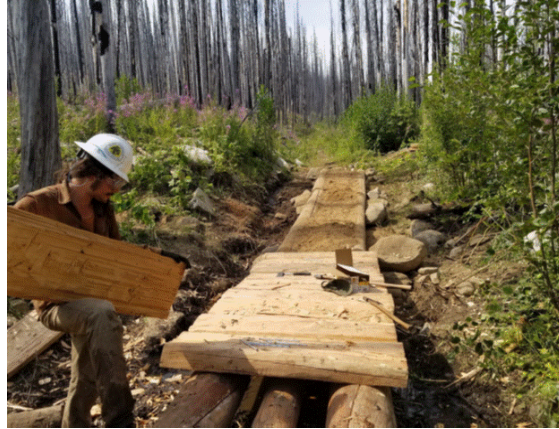
Pacific Northwest Trail Association Performance Trail Crew constructs a turnpike and puncheon bridge over a perennial seep and seasonal pond on East Deer Creek TR 6100-450.
