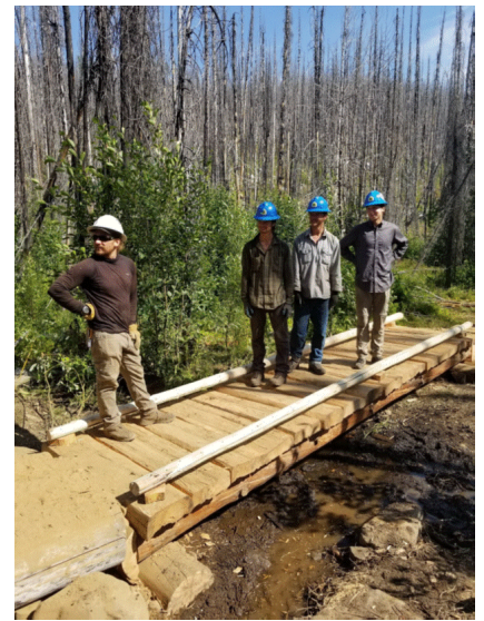
Pacific Northwest Trail Association Performance Trail Crew constructs a turnpike and puncheon bridge over a perennial seep and seasonal pond on East Deer Creek TR 6100-450.
