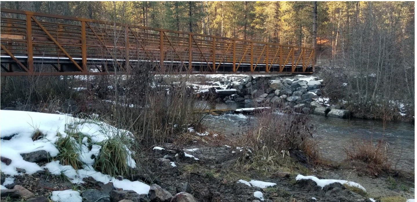
New Canyon Creek trail bridge over Sherman Creek in November 2021. The new bridge was extended 35 feet to allow the abutments to be located 10-20 feet outside of the channel and the stringers were elevated 5-6 feet to accommodate 100-year flood events.
