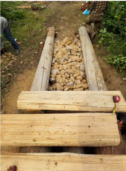
Pacific Northwest Trail Association Performance Trail Crew constructs a turnpike and puncheon bridge over a perennial seep and seasonal pond on East Deer Creek TR 6100-450.
