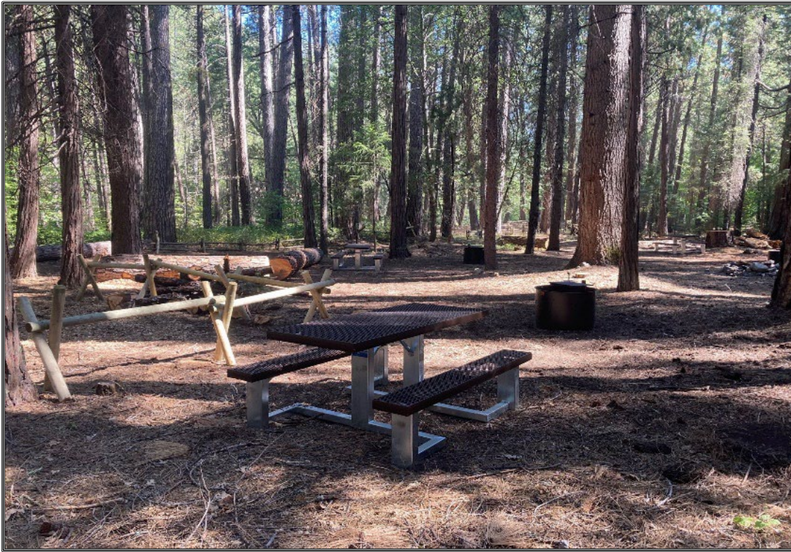
Highlands Lake Campground Picnic Table Installation
