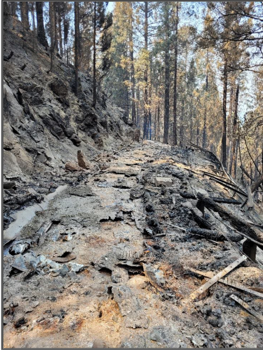
High intensity burned area and nearly 100% tree mortality. This was once the site of a historic wooden flume and critical water conveyance infrastructure which was completely consumed by the Caldor Fire.
