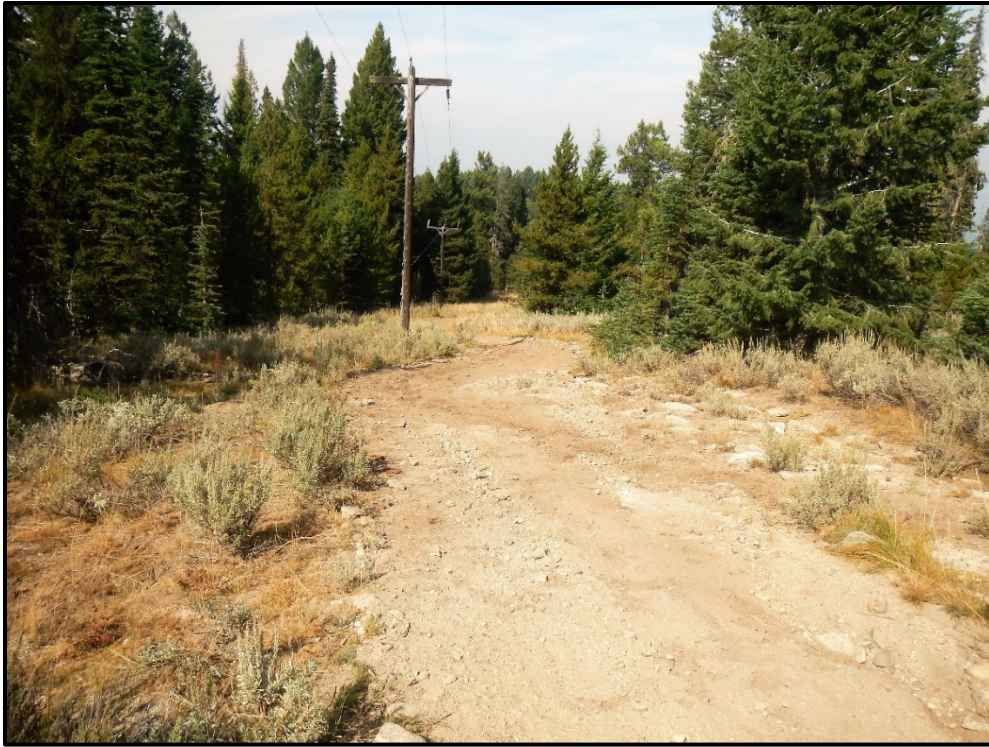
No Business Lookout Road Before
