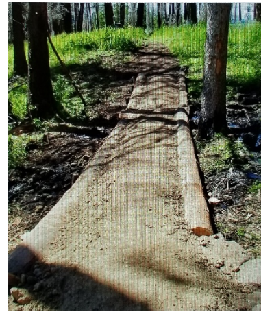
Center photo: Crew members fill turnpike with rock, gravel and soil using buckets, rope, and pulleys to minimize impacts to vegetation surrounding the seep.
