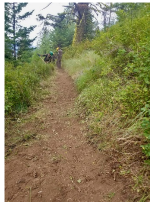
Left and center photos: NYC crew members start the process of brushing and reshaping the tread for improved cross drainage.
