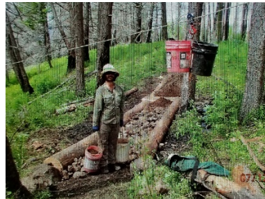
Left photo: PNTA crew member rolls retaining log into place for 45-foot-long turnpike.
