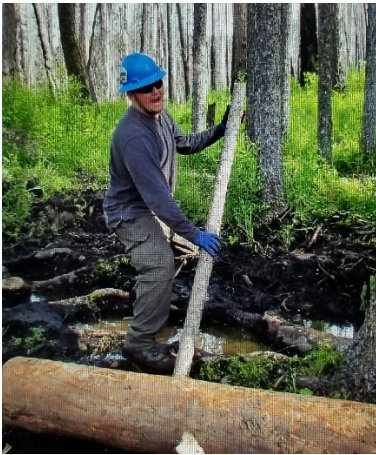
Left photo: PNTA crew member rolls retaining log into place for 45-foot-long turnpike.
