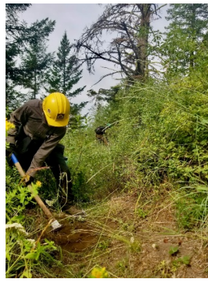
Left and center photos: NYC crew members start the process of brushing and reshaping the tread for improved cross drainage.
