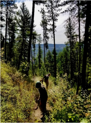
Left and center photos: NYC crew members start the process of brushing and reshaping the tread for improved cross drainage.
